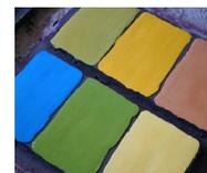
Oxide flooring : Cheap, variety of colours and cooling effect
